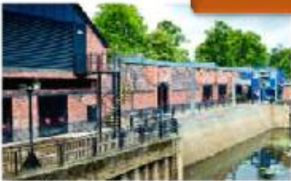
A flood defence wall
